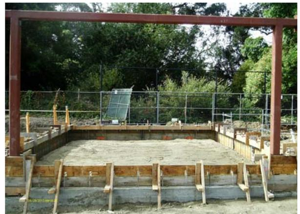
Storage Building moment frame up with formwork for slab
