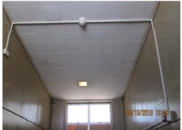
New Smoke Detector, Horn strobe, and J-box in Storage Room
