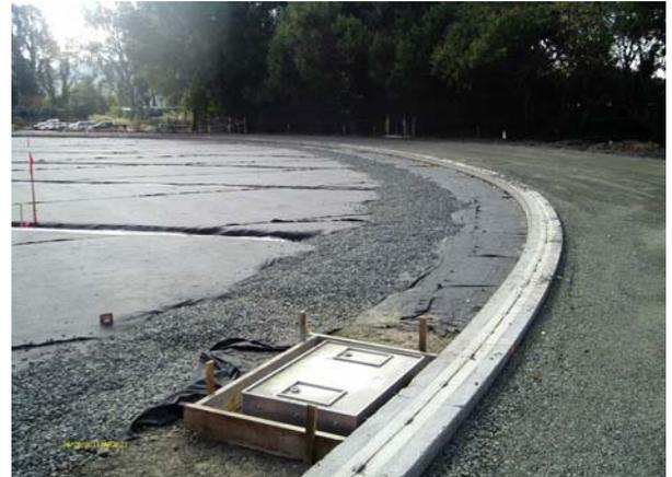
Perimeter drain, hose reel and AB placed on track
